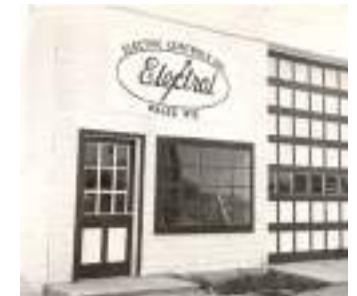
1959 - Wales, Wisconsin Garage
